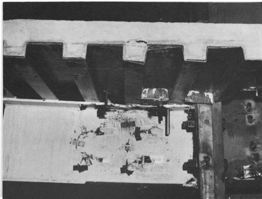
Fig. 58b Shearing of the Ribs and Local Buckling of the Top Flange of Test F2
