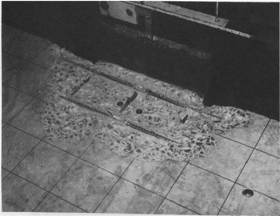
Fig. 41b B-66: Plan View of Failure Surface
