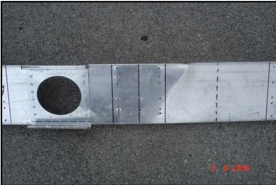
Figure C.2.4 Typical failure for specimens having reinforced (Scheme-“B”) circular web openings
