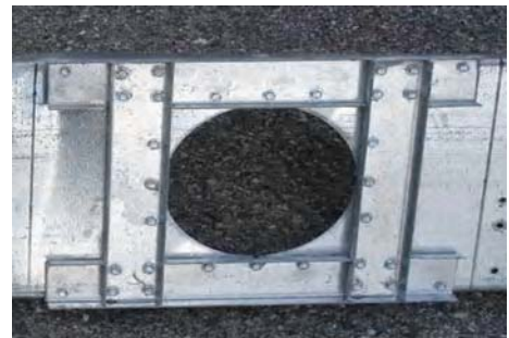
Figure 3.3 Vierendeel Reinforcement Scheme
