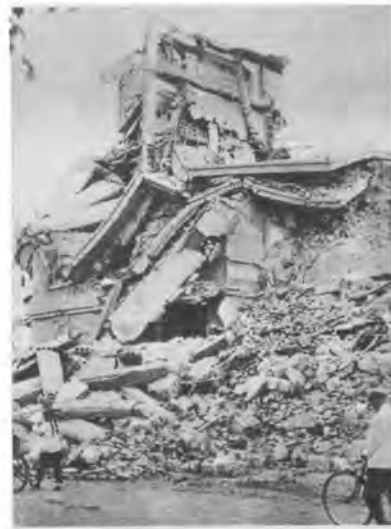
Fig. 2. A seven storey hospital building situated in I_0 = 11 area totally collapsed. However its underground chamber damaged very lightly.
