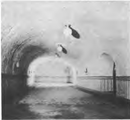
Fig. 3. An underground chamber stands still (only with very slight cracks) underneath severely damaged area of intensity I_0 = 11 .
