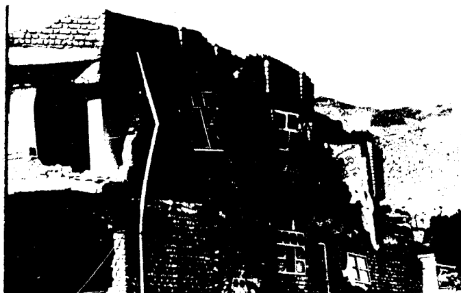
Figure-7 Picture of a Damaged Building
