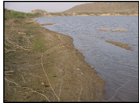
Figure 1g: Lateral spreading in the toe of Kaswati Dam
