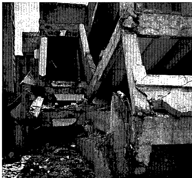
Fig. 2: Collapse of a four story structure in downtown Puebla in the zone of predicted maximum amplification
