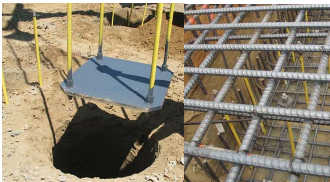
Fig. 1 RAP Uplift Bottom Assembly and Top Anchor
