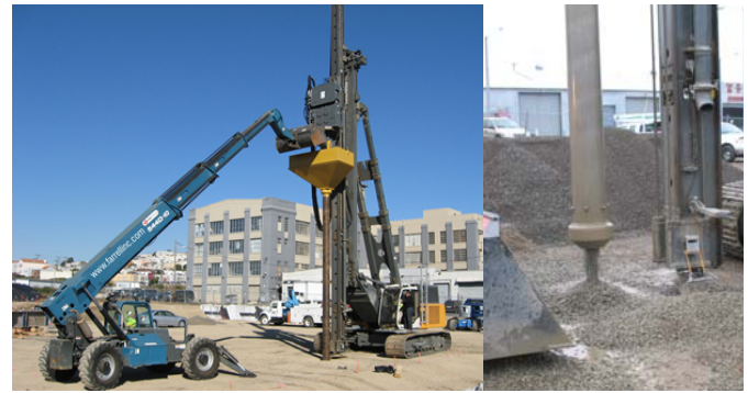
Fig. 2: Impact pier equipment with standard rammer head
