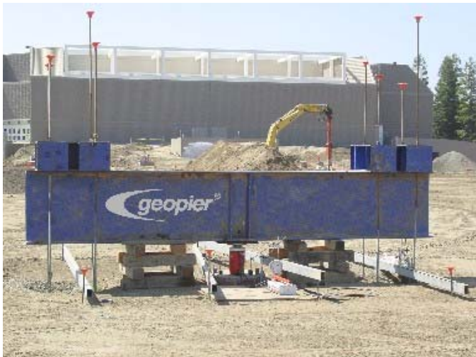
Fig.5. Section and Photo of RAP Modulus Test Set-up
