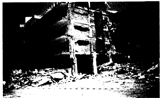
Fig. 4 Hotel collapse at "Valimitika", 15 June 1995.
