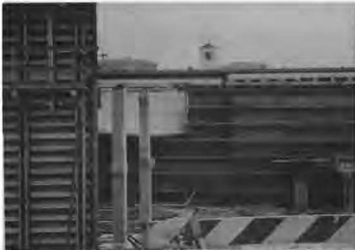
Figure 4 Union Station Gateway Construction Site Shoring
