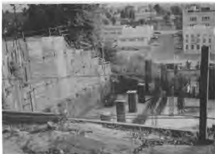
Figure 11 Construction Site West of Downtown Los Angeles
