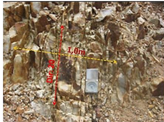
Figure 23. Broken zones in the rock at Nha Me
