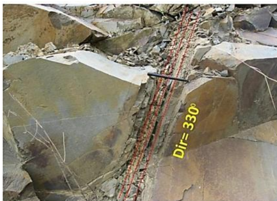
Figure 5. Broken zones in the rock at Ta Luong
