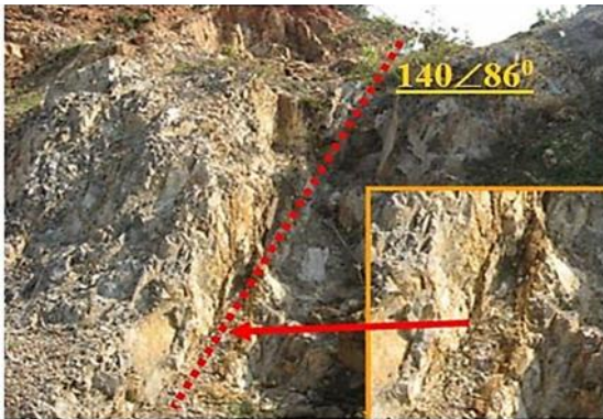
Figure 20. Broken zones in the rock at Vinh Hao
