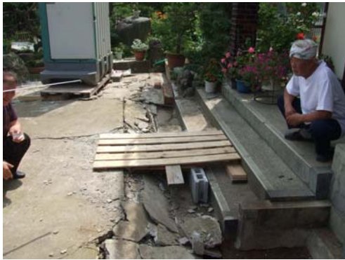
Photo 17. A settled house due to liquefaction though restored by short steel piles after the previous
