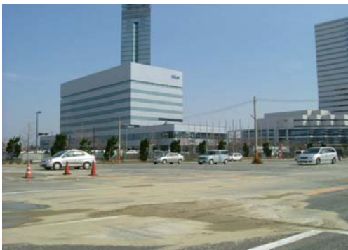
Photo 10. Boiled sand in Momochi-hama
