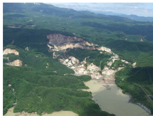
Photo 19. Biggest landslide at Aratozawa
