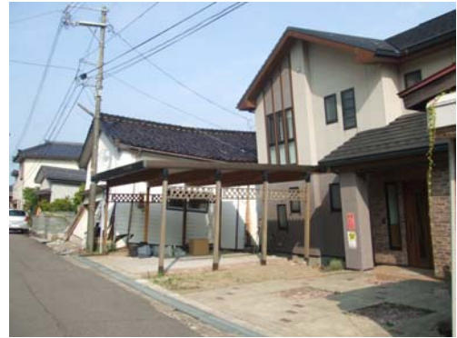
Photo 16. Damaged house due to liquefaction-induced flow in Yamamotodanchi district
