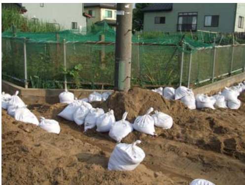
Photo 15. Erupted sand and a settled electric pole in Matsunami district
