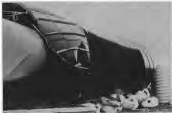
Fig.3. Collapse of Silo in Betsukai City.
