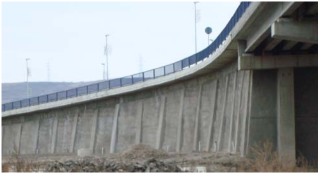
Fig. 2. Lateral view of the embankment.
