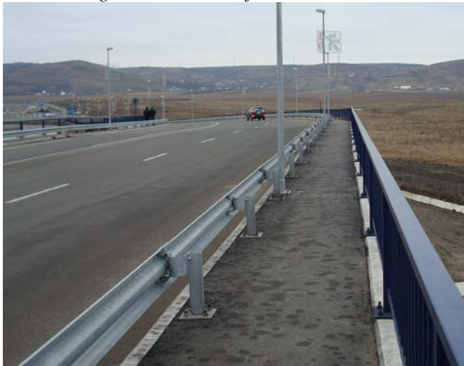
Fig. 3. Longitudinal view of the embankment.
