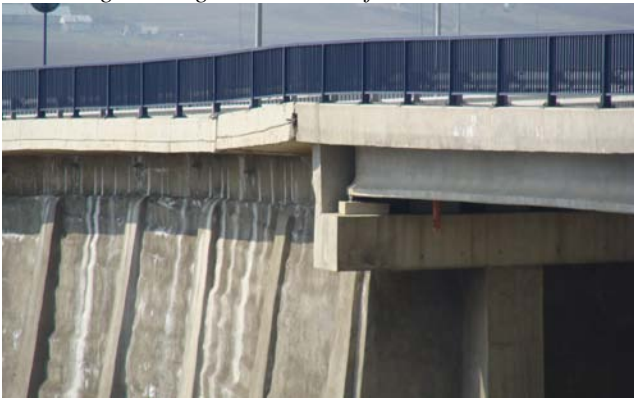
Fig.4. Zone between embankment - bridge.
