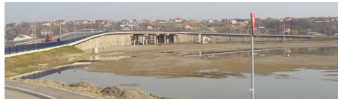
Fig. 1. General view of the embankment
