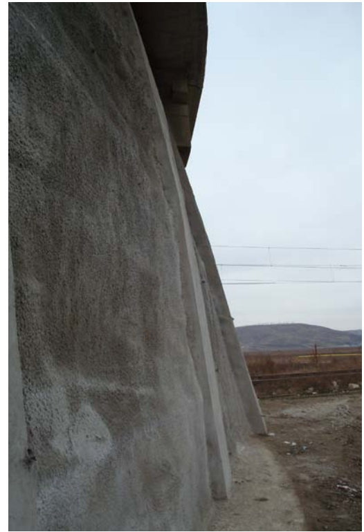
Fig. 5. Lateral view of the embankment.
