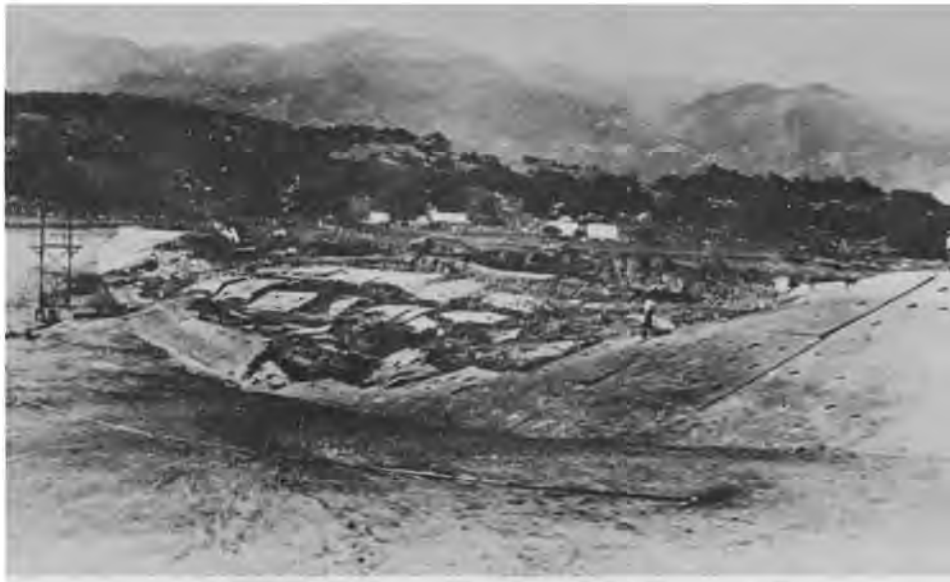
Fig. 3. Failure of Sheffield Dam in Santa Barbara Earthquake of 1925
