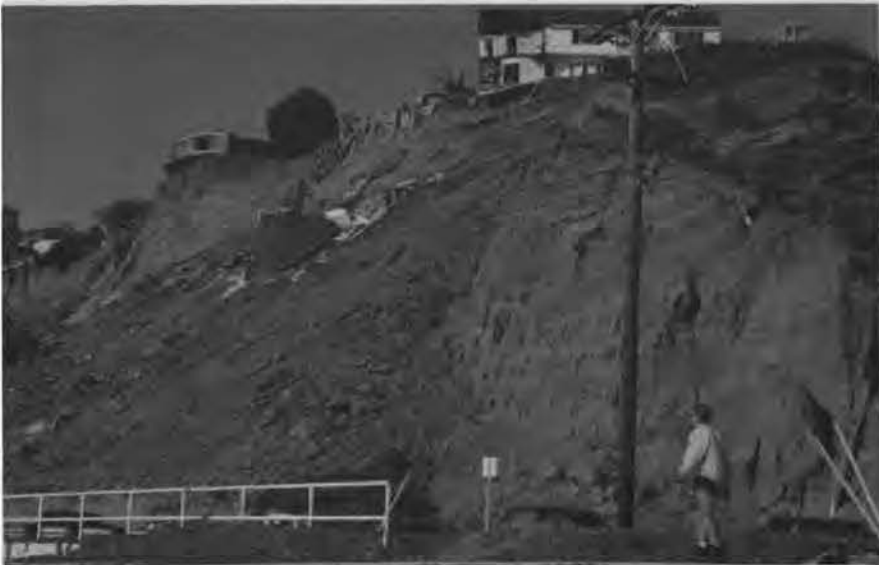
Fig. 10 Landslides in Santa Monica along the Pacific Coast Highway.
