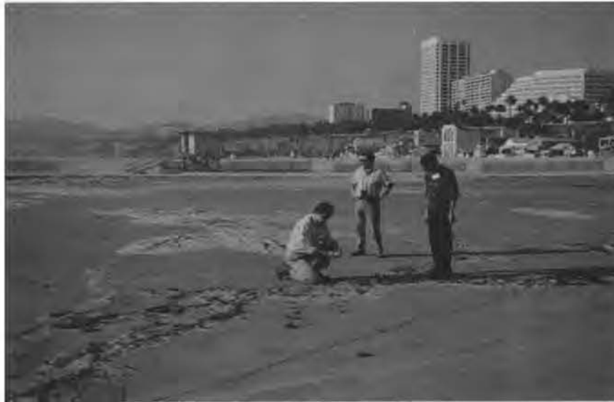
Fig. 5 Liquefied sand ejected from cracks in the pavement of the parking lot in Santa Monica Beach.
