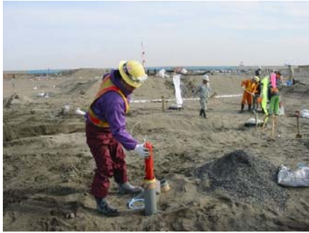
Photo 2 Charge Process of Explosive
