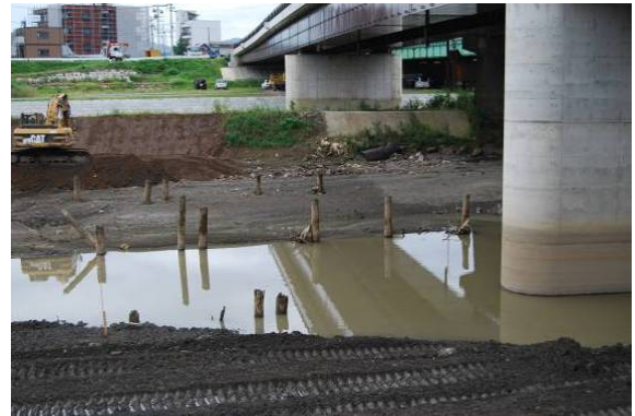
Photo 1. Former wood pile foundations near Kida Bridge
