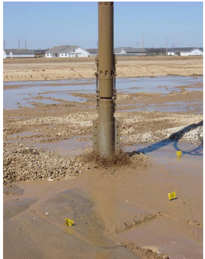
Fig. 5. Vibrocompaction in progress
