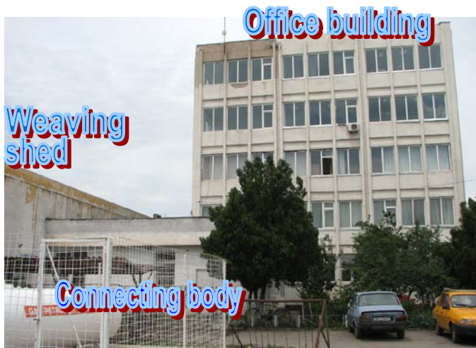
Fig. 1. General view of the complex of three buildings.
