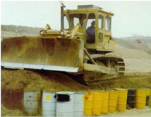
Fig. 4. Disposal of containerized liquid waste (Matasovic et al., 2006).
