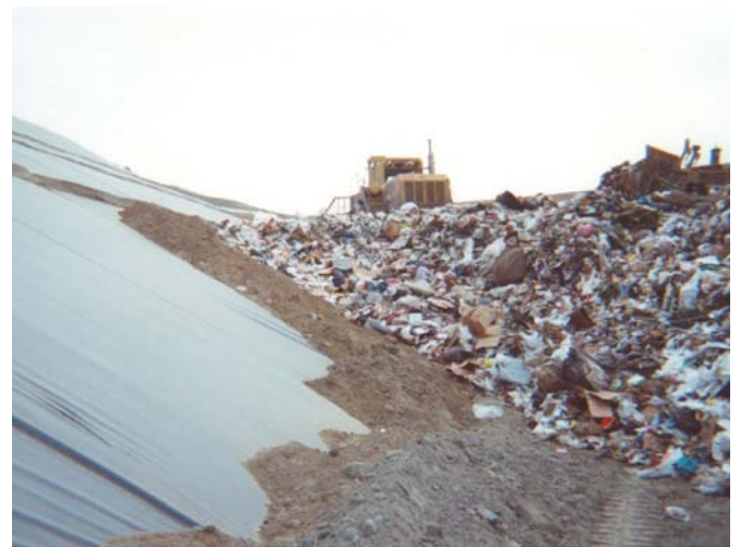
Fig. 2. MSW landfilling operation at a canyon landfill.
