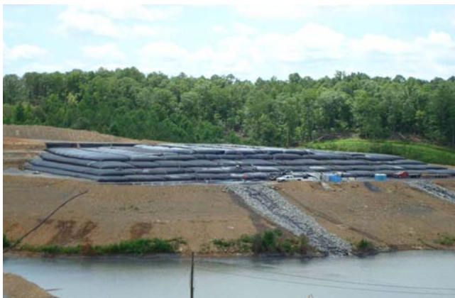
Fig 5. Sediment disposal using flat geotubes (Zhu et al., 2010).
