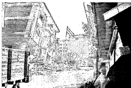
Fig. 15. Damage to building on Fabrika Cad.
