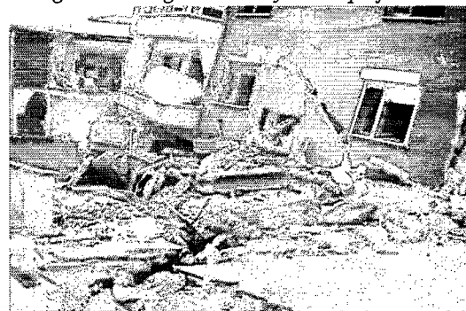
Fig. 8. Damage caused by soil liquefaction.
