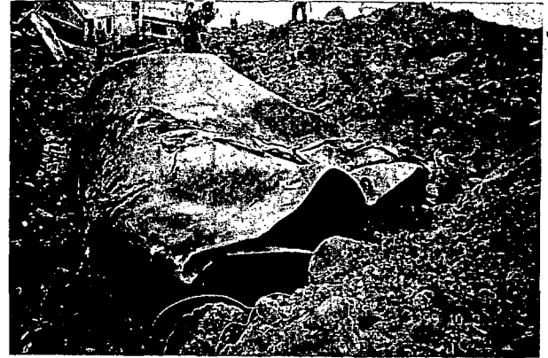
Photo 3 Damage to water conveyance pipe (Diameter: 2000mm).
