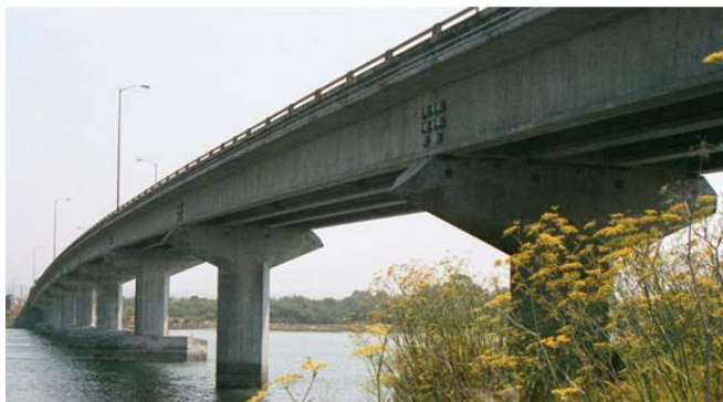
Figure 1. Humboldt Bay bridge (from Elgamal et al. 2008).
