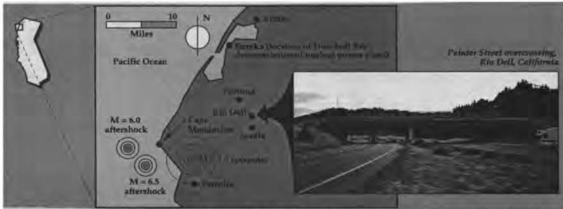
Figure 1: The Painter Street Bridge in Rio Dell, CA, and epicenters of the Petrolia Earthquakes of April 1992.
