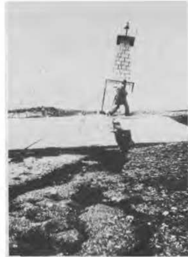
Fig. 5 Damage due to liquefaction: cracks in the soil and the concrete platform, sand outbursts, rotated lighthouse
