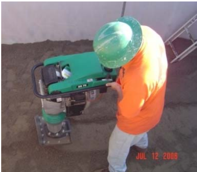
Fig. 8. Backfill compaction
