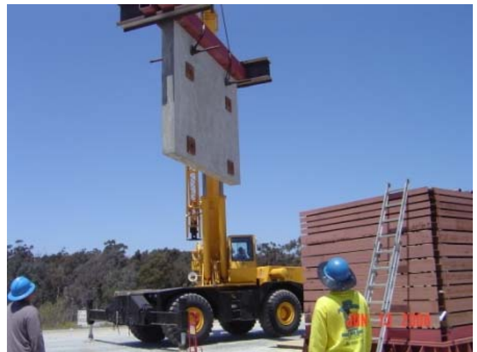
Fig. 5. Test wall section and supporting beam
