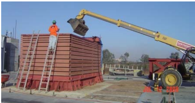
Fig. 7. Backfill placement
