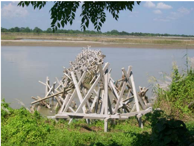
Fig. 4. Views of a typical porcupine field installed in the river
