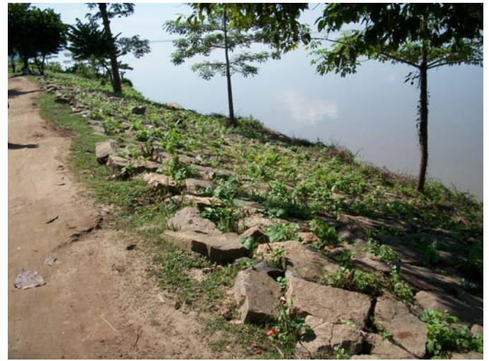
Fig. 12. Existing revetment riverbank protection at Palasbari
