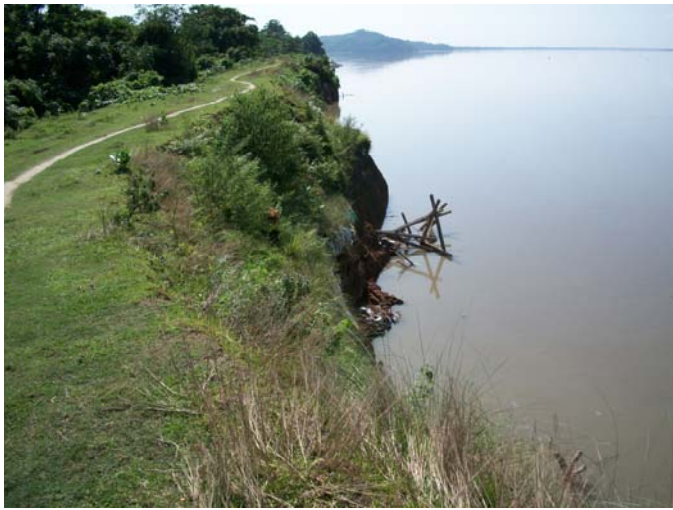
Fig. 11. Some views of riverbank erosion at Palasbari
