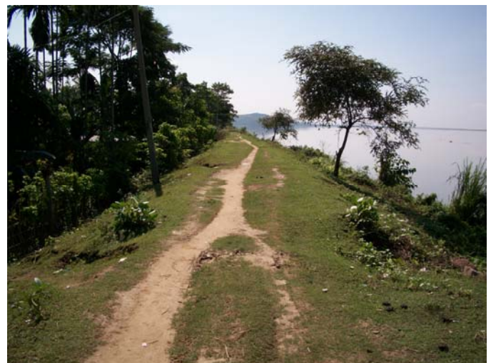
Fig.5. Views of existing embankments at Palasbari next to the Brahmaputra river
