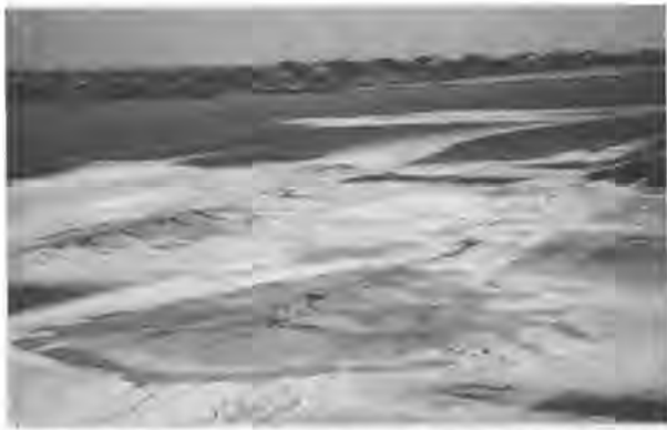
Fig. 16 Fissures and Exuded Boil Materials, Main Runway, Oakland International Airport
