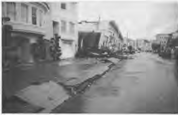
Fig. 6 Pavement Buckling Indicative of Lateral Compression; Marina District, San Francisco
