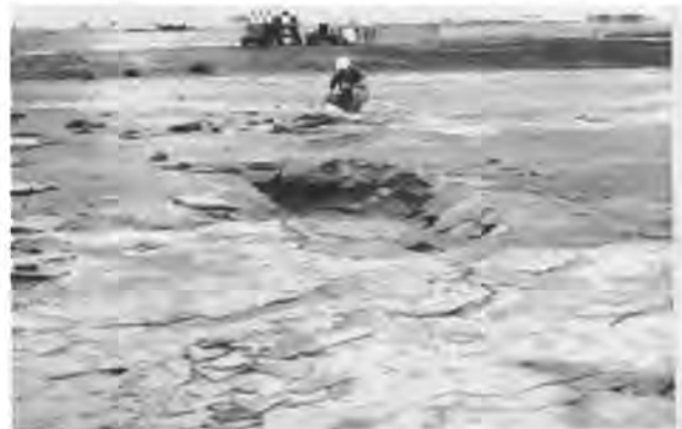
Fig. 15 Large Sand Boil and Sinkhole Adjacent to Runway at Alameda Naval Air Station
