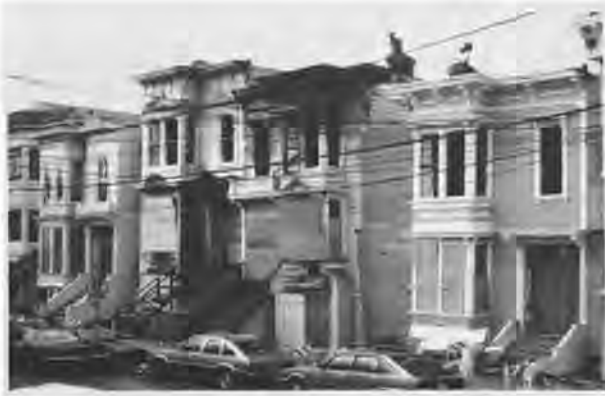
Fig. 10 Four Buildings on Shotwell near 18th Street Damaged by Liquefaction-Induced Foundation Displacements in the Loma Prieta Earthquake
