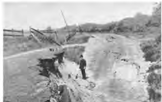
Fig. 19 Apparent Massive Lateral Spreading and Settlement at the Edge of the Salinas River, Near Spreckels, After the 1906 San Francisco Earthquake [Lawson et al., 1908]
