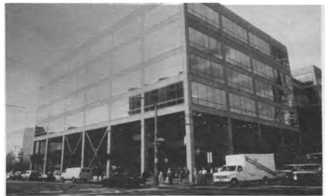
Fig. 11 Retrofit of New Reinforced Concrete Building
