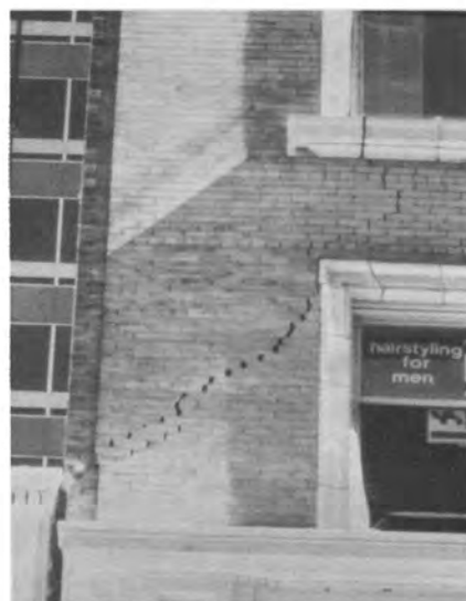
Fig. 17 Pounding Damage
