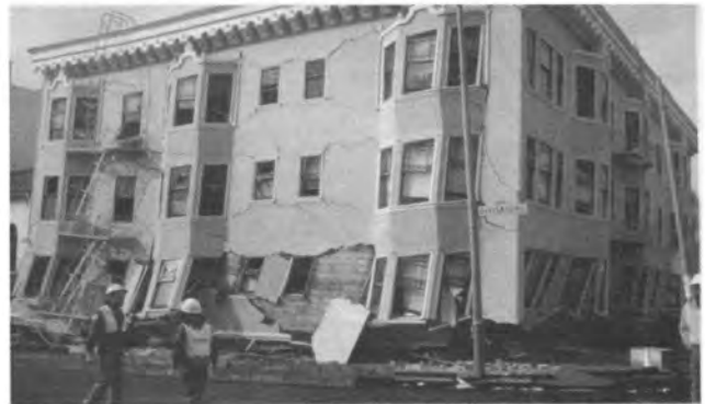
Fig. 5 Collapse of Apartment in Marina District
