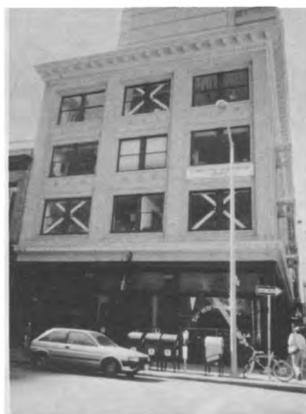
Fig. 15 Retrofit URM Building with Steel Braces
