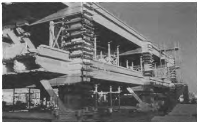
Fig. 26 Cypress Street Test Structure
