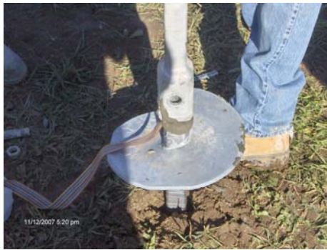
Fig.7. Typical preparation of lead section – extension connection
