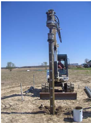
Fig. 8. FRP-G-HSP installation (internal SS175 shaft – external FRP 3m tube).
