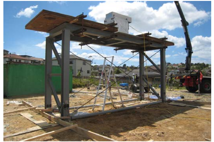
Figure 12 Shallow foundation test structure with shaker in place and additional weight added.
