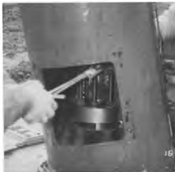
Fig. 7 Prestressing force tensioning.
