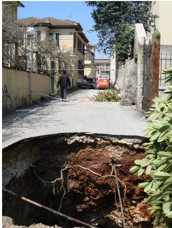
Fig. 12. Hole formed at L'Aquila city after the Apr 6 2009 earthquake and caused by the opening at ground surface of a buried natural cavity. Courtesy of F. Benedettini.
