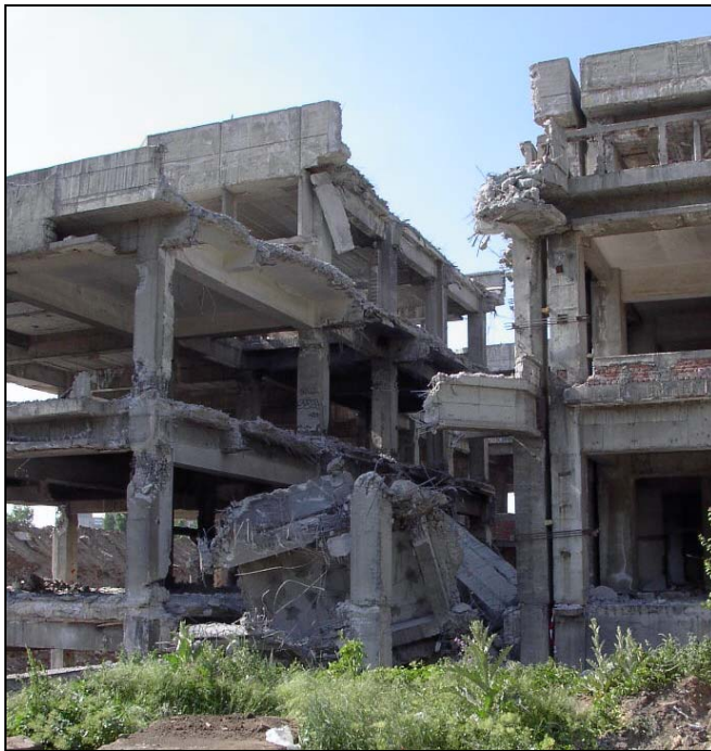
Fig. 43. View of the lateral wing before the demolition.
