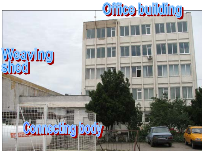
Fig. 28. General view of the complex of three buildings.
