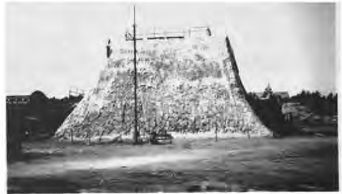
Figure 3. General View of Retaining Wall
