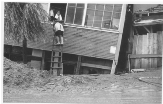
Fig. 1. Liquefaction-induced subsidence of building during the 1964 Niigata earthquake (Department of Civil Engg, University of Tokyo).
