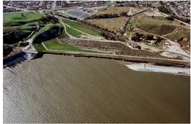
Fig.1 –San Fernando dam-dam view
