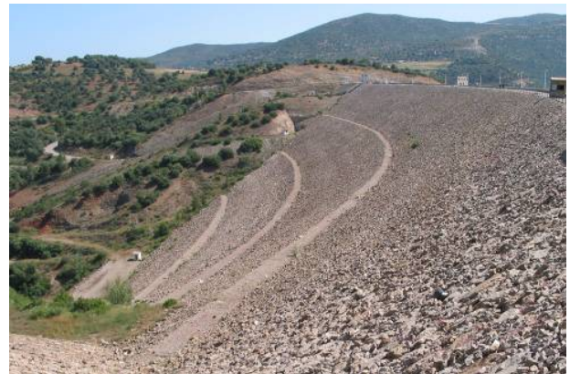
Fig. .5 Keddara dam-downstream view
