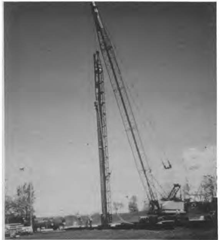
FIGURE 14 - Pile Driver at Northwestern Site
