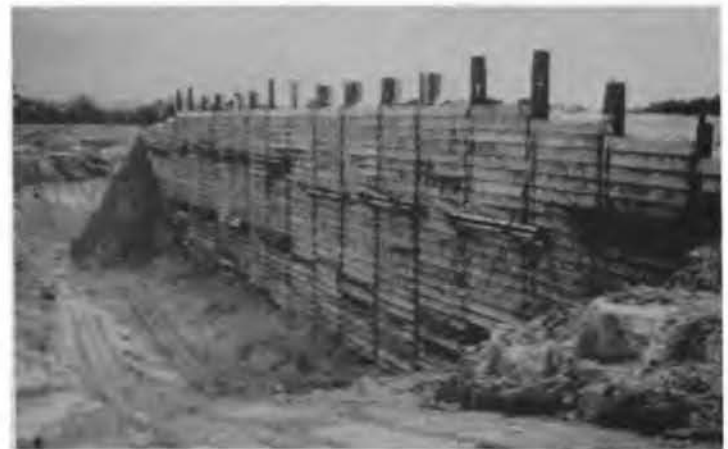
FIGURE 7 - Tied-Back Retaining Wall Experiment
