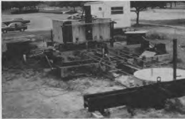
FIGURE 12 - Drilled Pier, Lateral Load Test
