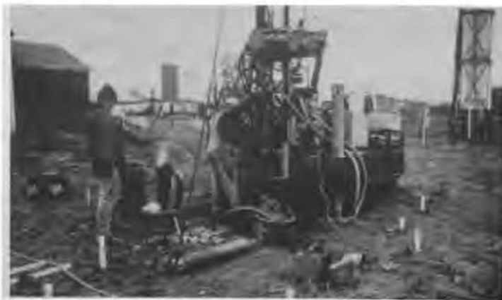
FIGURE 16 - Installation of Pneumatic Piezometers at UMASS Site
