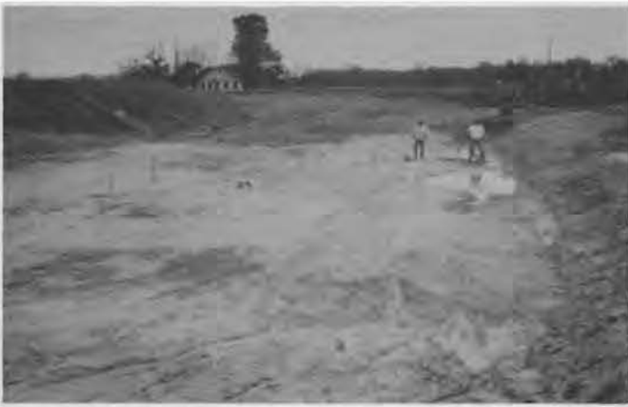
FIGURE 8 - Sand Site for Spread Footing Tests
