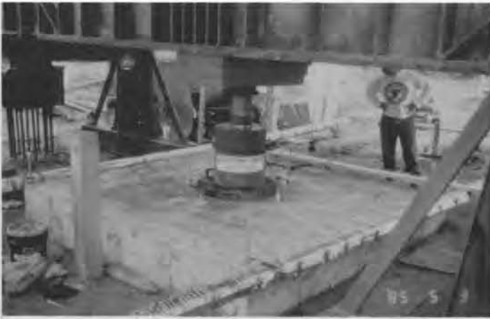
FIGURE 9 - Load Test on Spread Footing, TAMU
