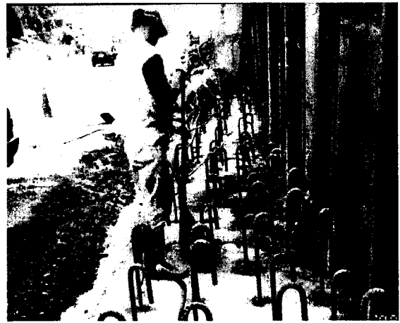
Fig. 4. Shearing reinforcement at construction joint.
