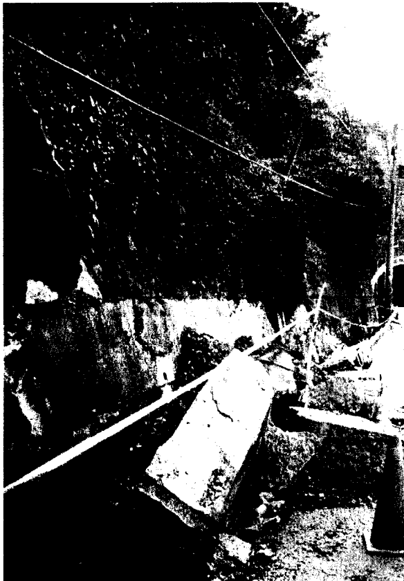
Fig. 3. Sliding and falling of gravity wall.
