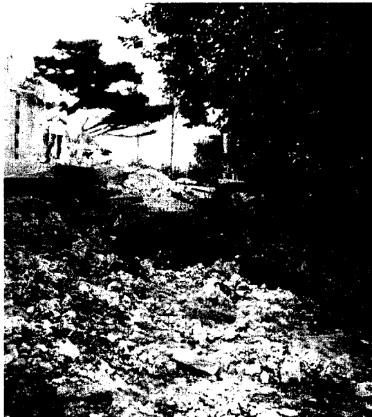
Fig. 14. Pavement and backfill damaged.
