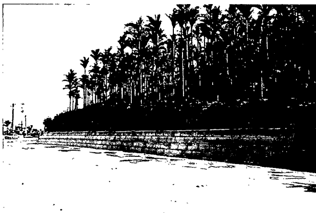
Fig. 7. Repaired retaining wall.
