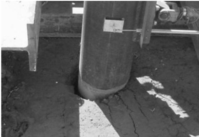
Fig. 28 Photograph of a gap formation behind the pile (the pile is deflected laterally to the right and the gap is formed on the left of the pile in the photo) (Snyder, 2004)
