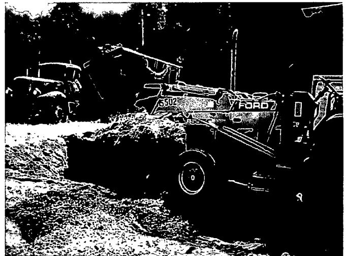
Fig. 2 – Crushed Rock Dumped into Test Trench
