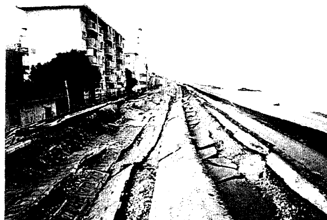
Fig. 1. Distorted shape of Yodo River dike (by Fudo Construction Company).
