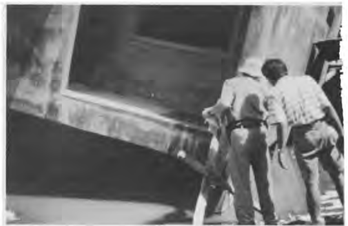
Photo 7 Three-storied building settled by 2 meters
