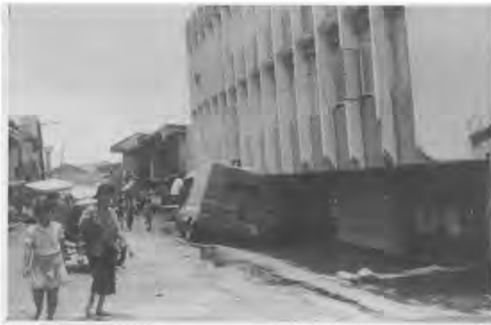
Photo 6 Damage in Fernandez St. - building is supported by a trapped van
