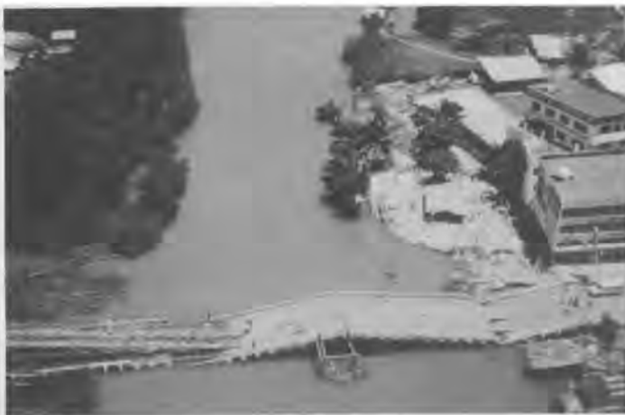
Photo 4 Collapsed bridge and narrowed river
