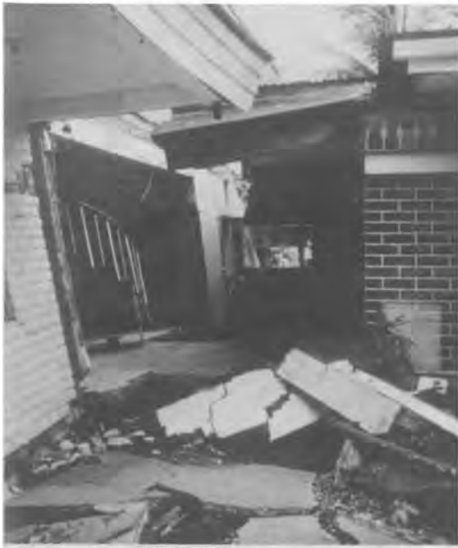
Photo 12 Damage to house in sliding area
