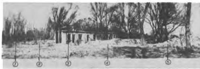
Fig.3.5 Houses damaged intermittently; (1),(3) stood still; (2),(4),(5) crushed down
