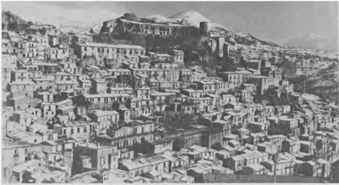
Fig. 10. View of the old section of Muro Lucano. Note stripe of heavy damage running from top left to bottom center of the picture.
