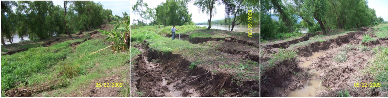
Figure 9 – Multiple views of severe lateral spreading between levees and river [06/22/2009, 10:25AM, N15.391266, W87.845191].
