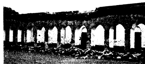
Photo 5 Madarsa Building, Darbhanga (failure of arches)
