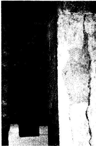
Photo 3 Surgical ward, Darbhanga (Cracks in r.c. column)
