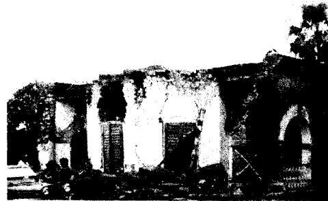
Photo 3 Land Mortgage Building, Darbhanga (Failure of front arches, walls and roof)
