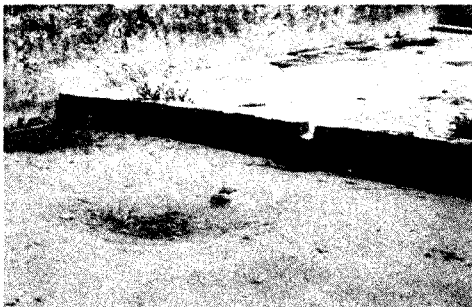
Photo 10 Jail Building, Darbhanga (Circular patch of sand left over after liquefaction)
