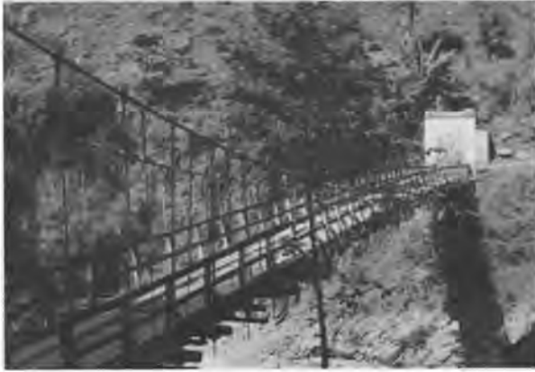
FIG. 14 Old Suspension Bridge Near Tashiding Bridge, Sikkim (no damage).
