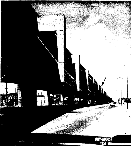
Figure 9 - View looking north at the east side of the newly-completed double-deck Cypress Viaduct from Sixteenth Street in June, 1957. The Fourteenth Street on-ramp is cantilevered from the main support bents at left foreground. The October 1989 collapse preceded south to Bent 62, indicated by arrow (Calif. Highways & Public Works).
