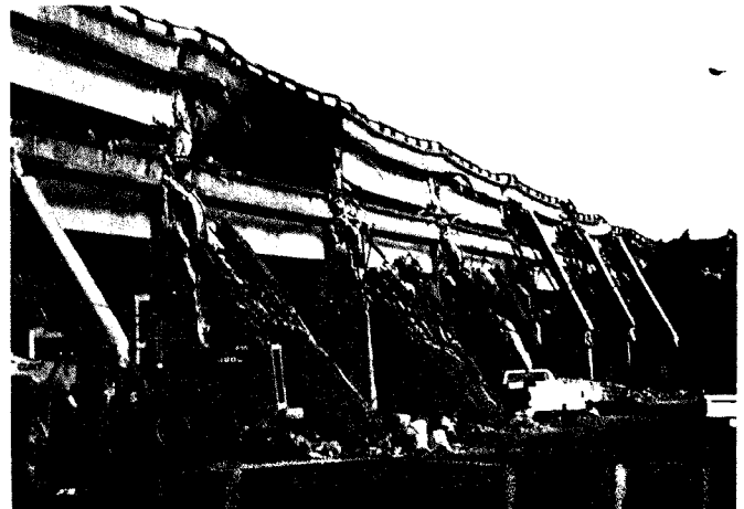
Figure 18 Lower - Photograph of the dominant failure mode sketched above. Dark area is from diesel fire which broke out shortly following the collapse.
