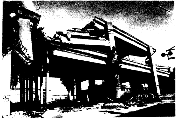
Figure 25 Upper - View of lone surviving section of the Cypress Viaduct, a skewed railroad crossing at Thirty-second Street. One truck (arrow) and two cars found sanctuary here. The crossing was supported on a 3-column base bent with a large pedestal area due to the skew.
