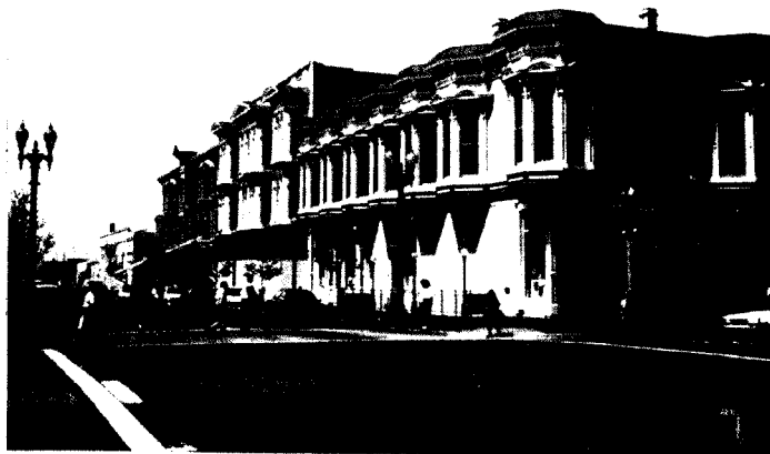
Figure 2 - The Wilcox Building on the northwest corner of 9th and Broadway in downtown Oakland. Originally built in 1865 on the Merritt Sands, it has withstood every earthquake since that time.
