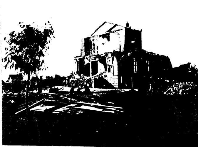
Figure 1 - Remains of Alameda County Courthouse in San Leandro following the M 6.8 Hayward Earthquake on October 21, 1868. The Courthouse was then moved to Oakland because its structures fared much better in both the 1865 and 1868 earthquakes (Oakland Public Library).
