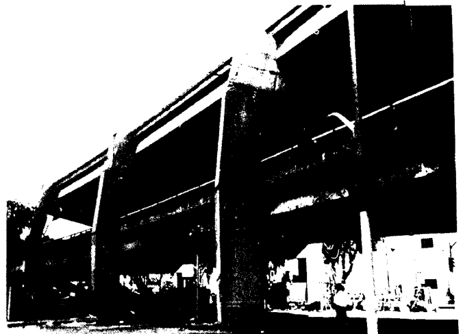
Figure 22 - Ground view of Grand Avenue overcrossing partial collapse, as seen from the west side of the viaduct. Note how the doubly hinged upper columns simply rotated at their hinges.
