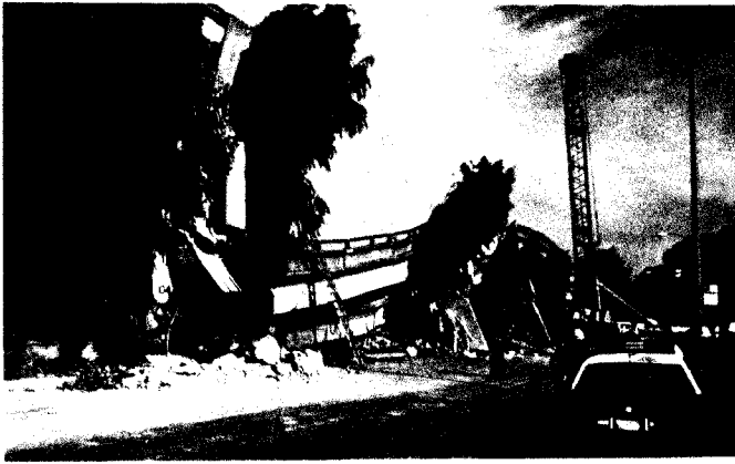
Figure 26 - Between Bents 104 and 106, both decks of the Cypress fell to the ground, the only location where total collapse occurred. In this area the decks collapsed asymmetrically, with the upper deck falling to the east of the lower. This suggests different parts of the appurtenant supporting bents failed in differing manners, or at slightly different times (and motion phases would not be aligned). In this area, the lower supporting columns rotated outward, about their respective basal hinges.
