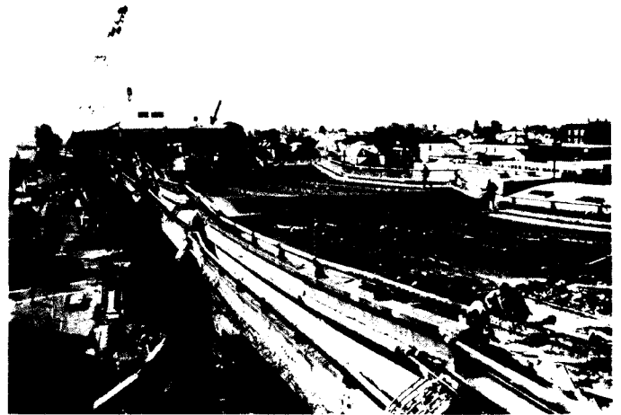
Figure 12 - Overview of Cypress Viaduct collapse looking southerly, towards the unfailed portion, at Bent 62 (arrow). The northern half of the double-decked structure experienced a partial collapse of the upper deck onto the lower deck.
