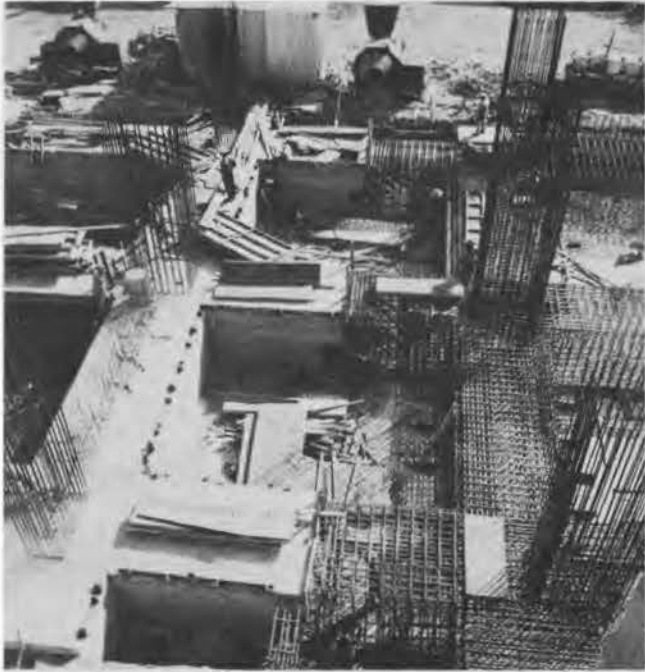
Fig. 7. Construction Joints - Longitudinal Ribs
