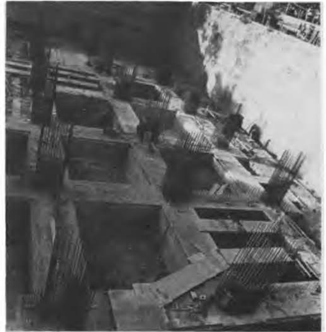
Fig. 8. View of Complete Mat Foundation.
